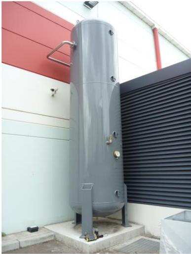
A pressure vessel is a container that holds either gasses or liquids and is subject to internal or external pressure. It includes interconnecting parts and components, valves, gauges, and other fittings up to the first point of connection to the connection piping.
